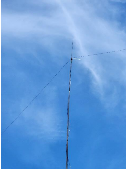
10-40m OFC Dipole deployed on the 7m Sotabeam mast
