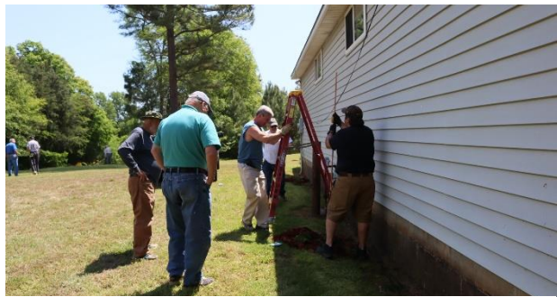
Club Members prepare to drive another ground rod
