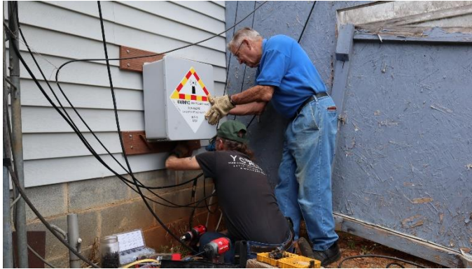
Wayne KD4RDP and Tim K6FNV install the grounding enclosure
