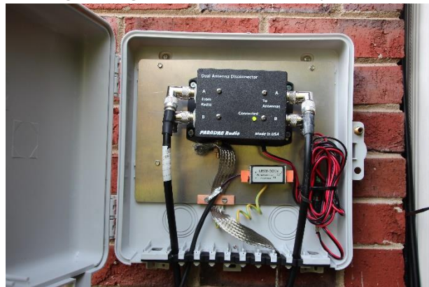
Paradan Radio dual disconnect in DXE enclosure
